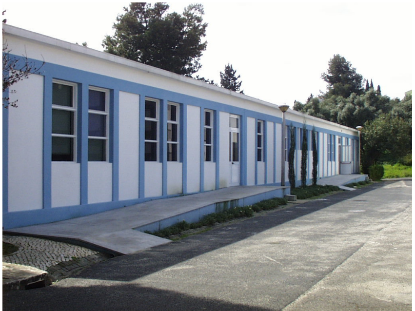
Outside view of Building for Cryogenic Techniques
